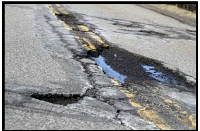
Poor Road Surface Rating
